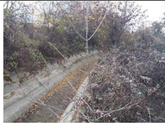
Existing canal downstream intake K36
