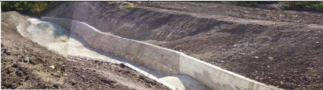
Lateral Spillway: Sky jump and stilling basin
