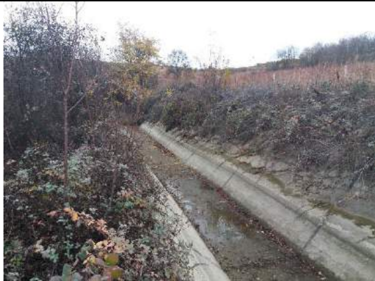
Existing canal at intake K36
