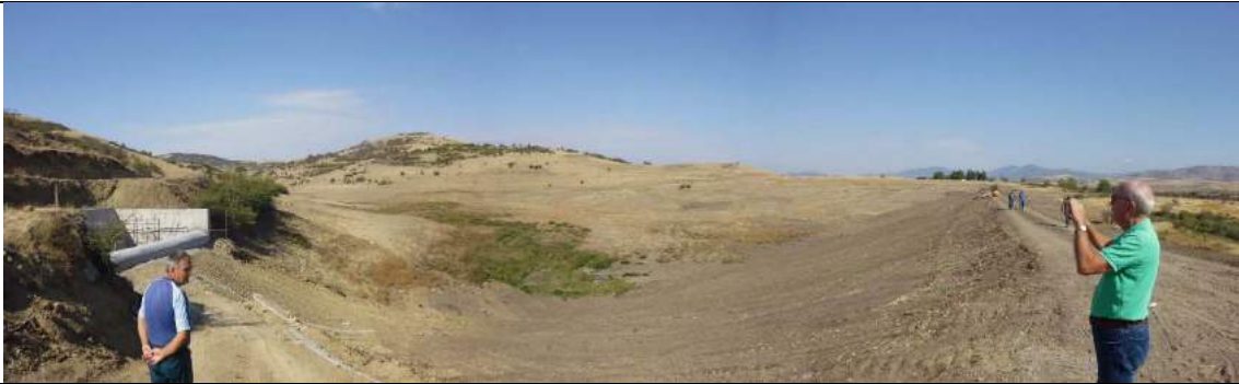
New lateral spillway, reservoir and Pishica Dam
