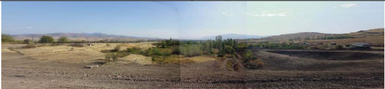
Downstream Pishica dam. Irrigation canal begin from irrigation outlet.
