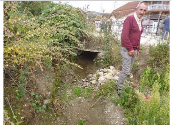
Secondary canal to be lined
