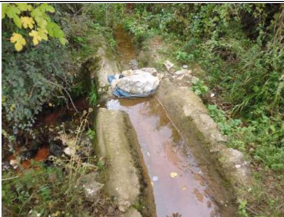
Secondary canal to be rehabilitated
