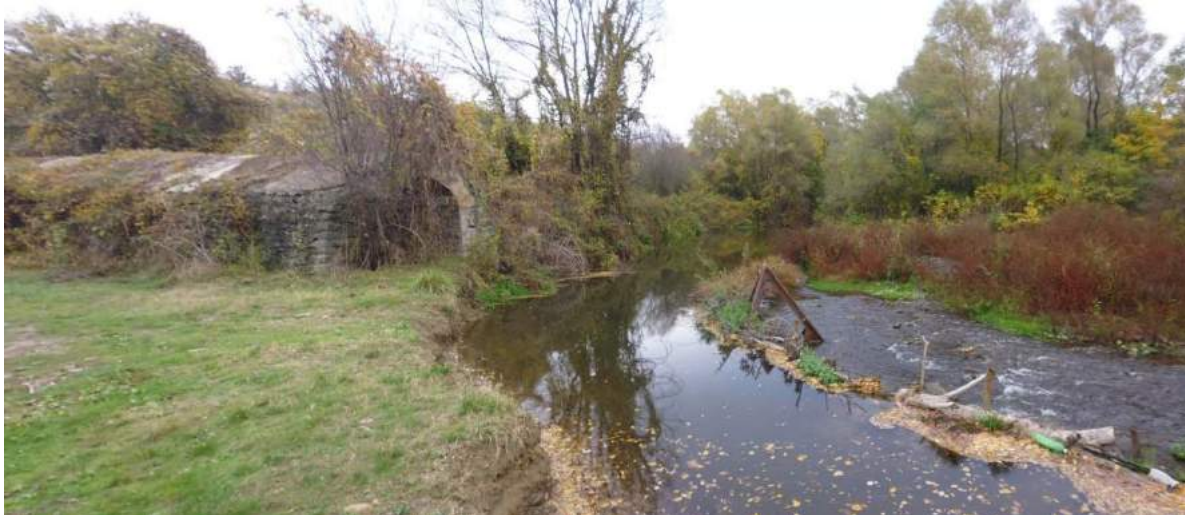
Intake at Kriva Reka and beginning of main canal
