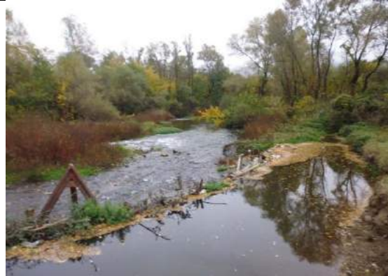
Main canal beginning from intake
