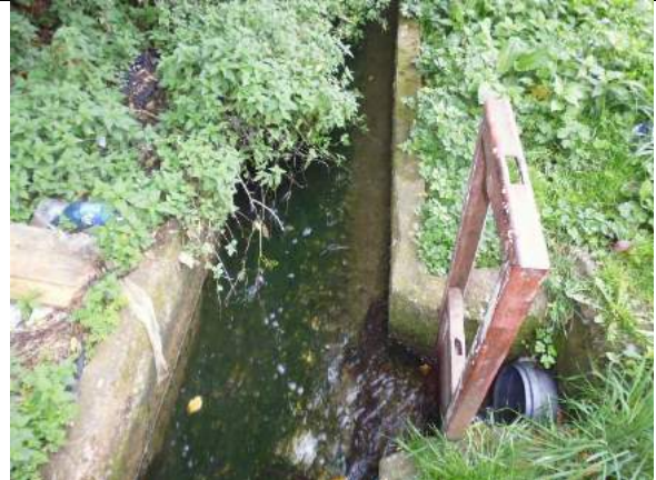
Main canal and field diversion
